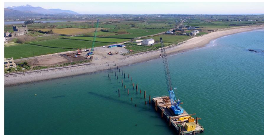
**Greenore** – A cofferdam was installed using A-Z sheet piles and our Movax excavator mounted vibro hammer with a steel ground gate to keep the pile line within tolerance. The Main contractor formed a stone platform which allowed us to utilise our ABI 14/17 piling rig to close in the cofferdam.
