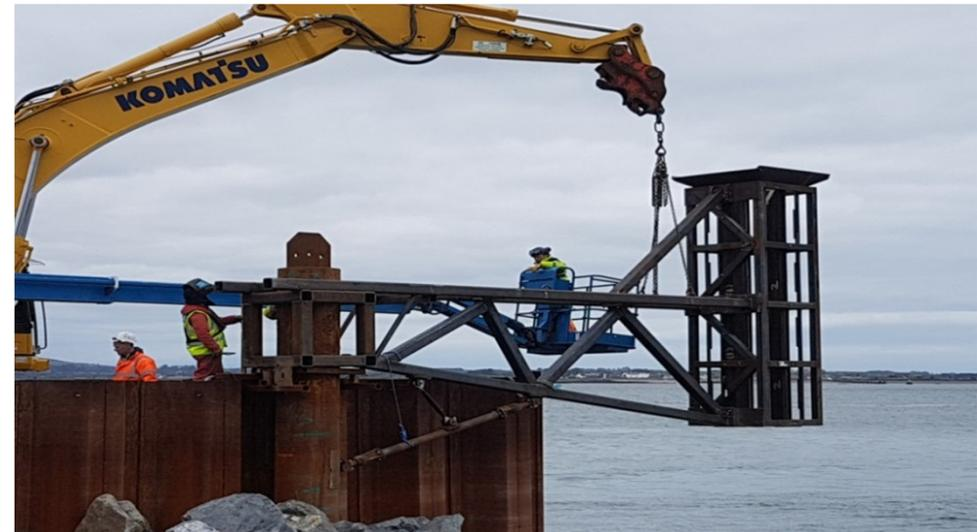
Gate installed onto last tube pile of cofferdam
