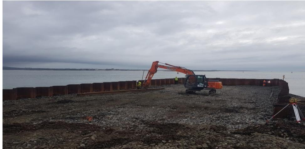
Cofferdam filled to provide working platform
