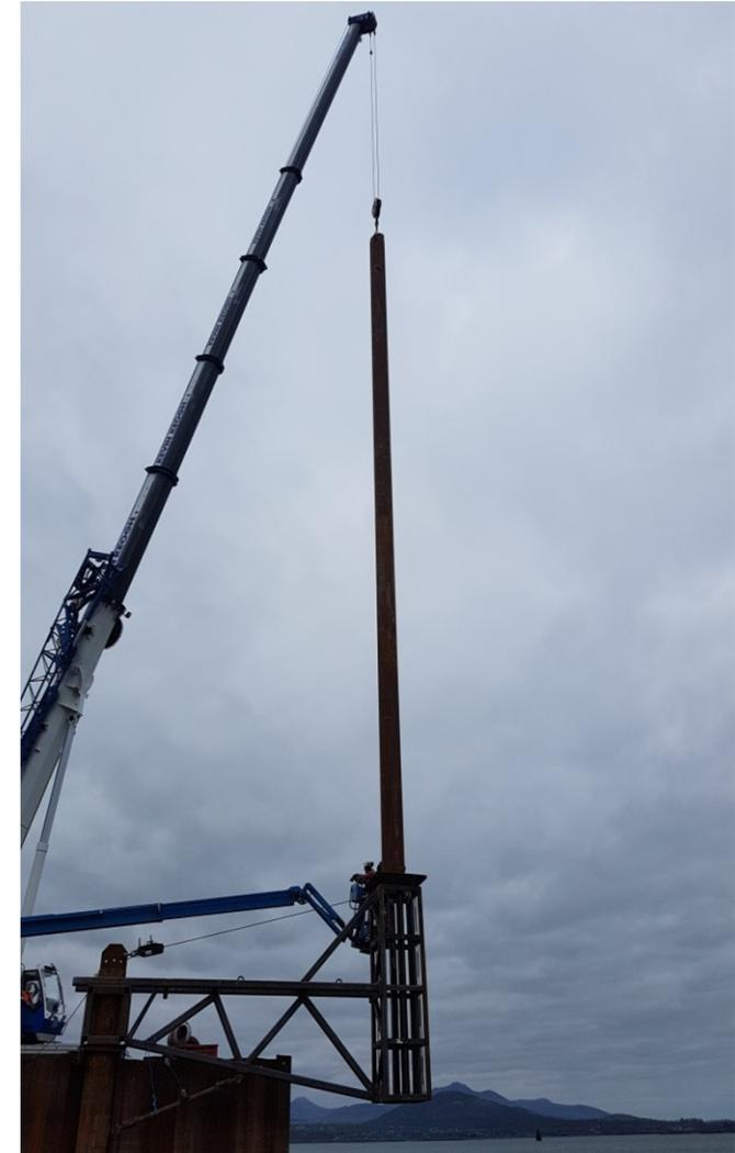
130t Crane installs pile into position
