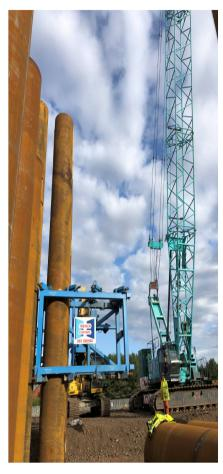
Once the combi tubes were pitched into position and are to vibro refusal, Trench control team impacted these tubes using CG300 impact hammer to initial refusal level. The main contractor then proceeded to core out the internals of each tube removing the debris from inside the tubes. TCL would then return to the cored tube and impact again to the design depth required.
