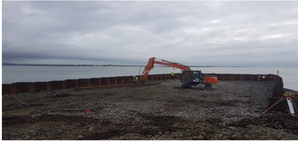
Cofferdam filled to provide working platform
