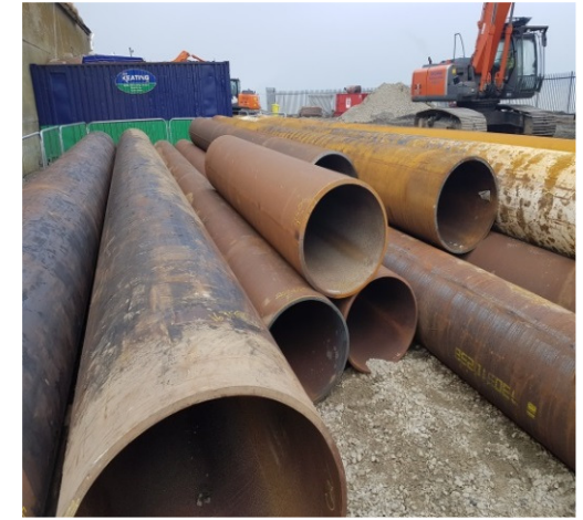
Steel tube fender piles spliced
