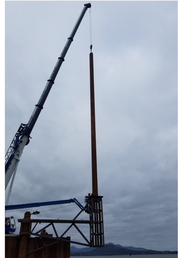
130t Crane installs pile into position
