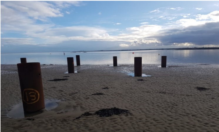
Impacted to cut off height
