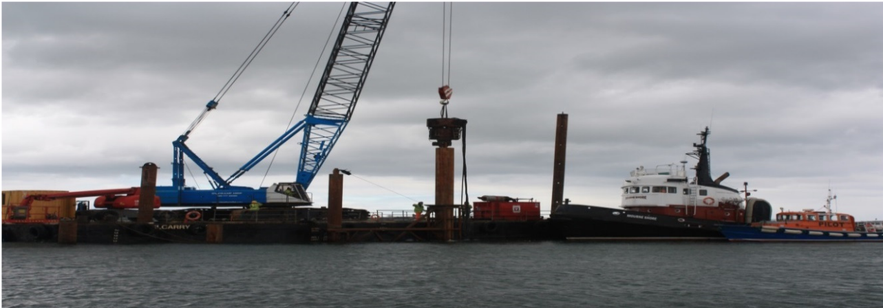
Spud barge manoeuvred into place for final fender pile
