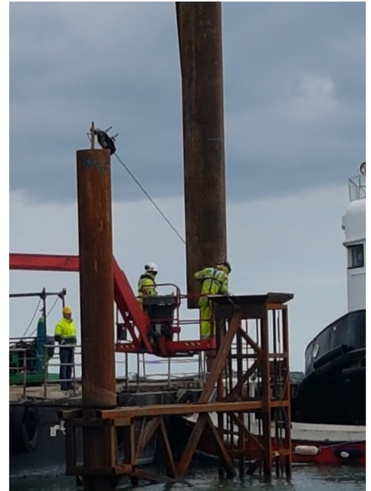
Fender pile installed at high tide
