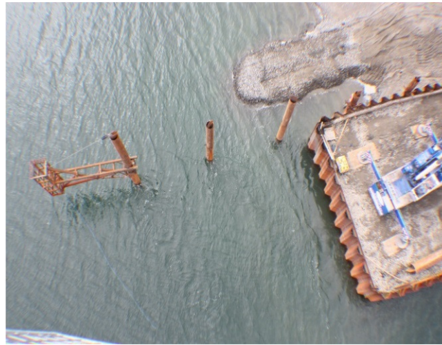
Aerial view of fender pile set up
