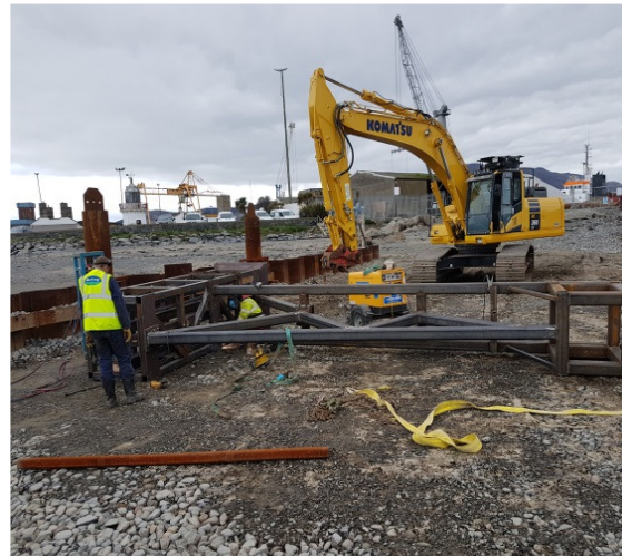
Gate assembled on site
