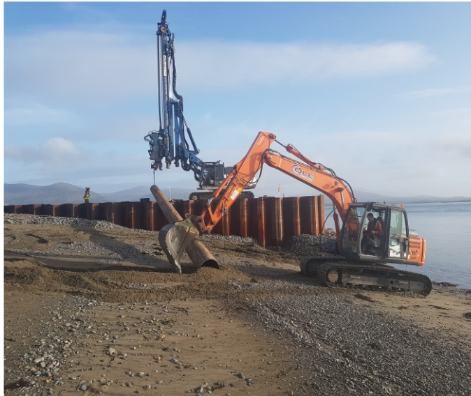
Spliced tube for installation
