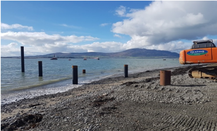
Low tide allowed piles to be installed from beach
