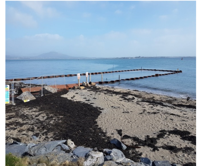
Cofferdam flooded with tide
