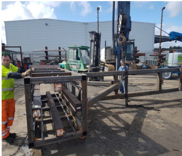
Prefabricated piling gate
