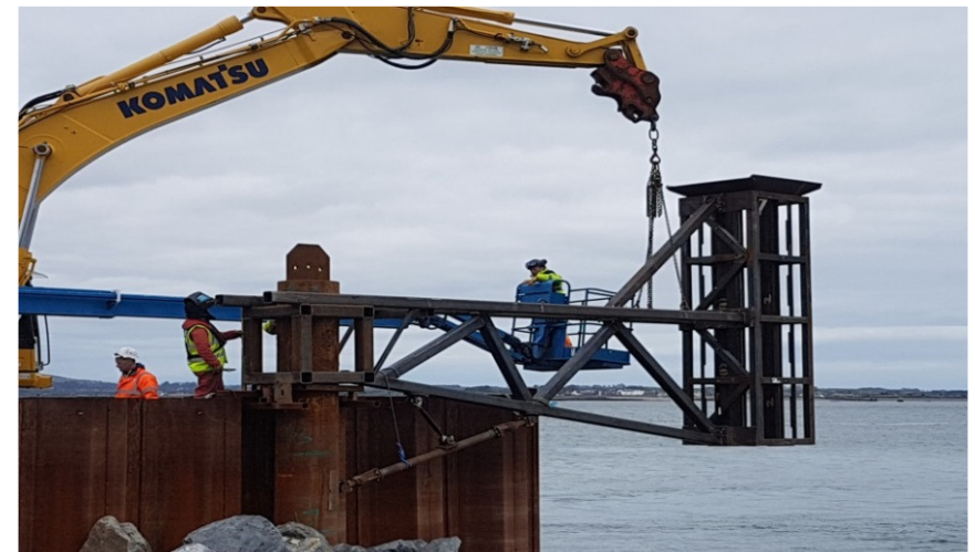
Gate installed onto last tube pile of cofferdam
