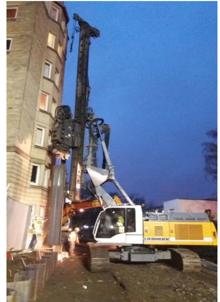
Leader Rig with less than 0.5m clearance
