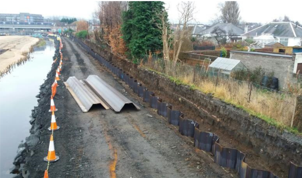
Temporary stoned platform to allow installation at bank edge
