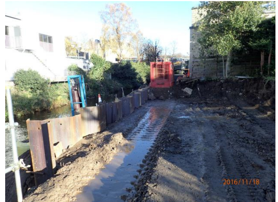
Pile line running close to the rear of existing buildings
