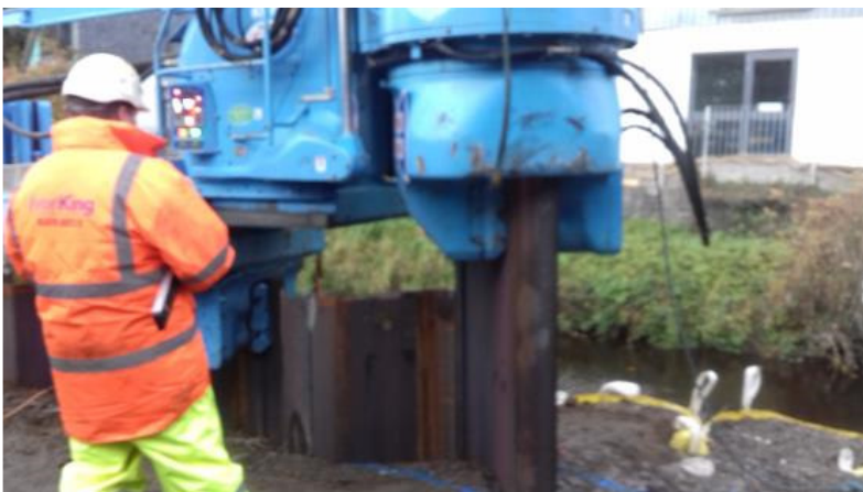
Pile Press reaching design depth
