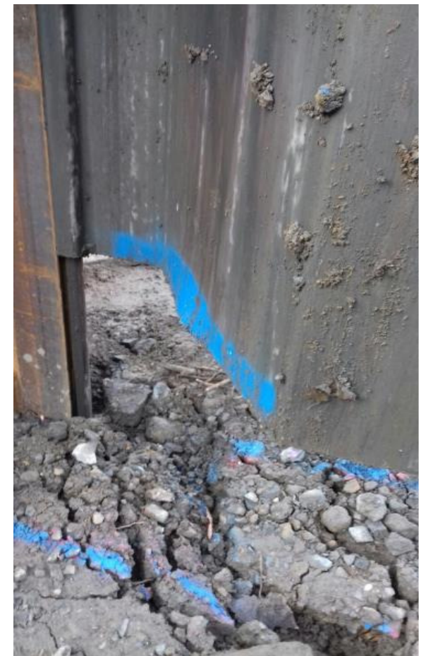
Still ground causing damage to pile toe
