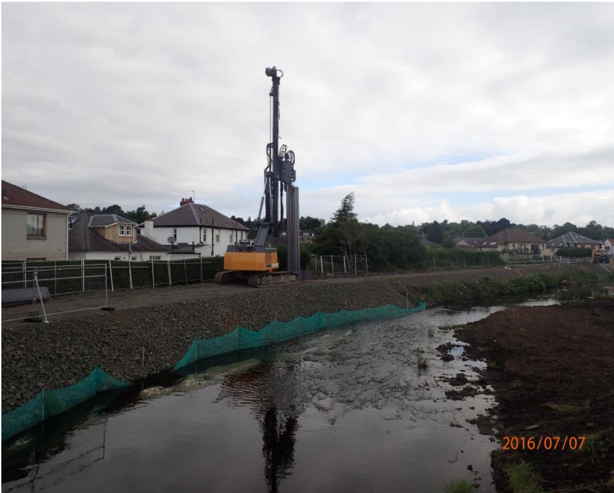
Narrow platform built into the Leith river to allow leader rig access to all areas
