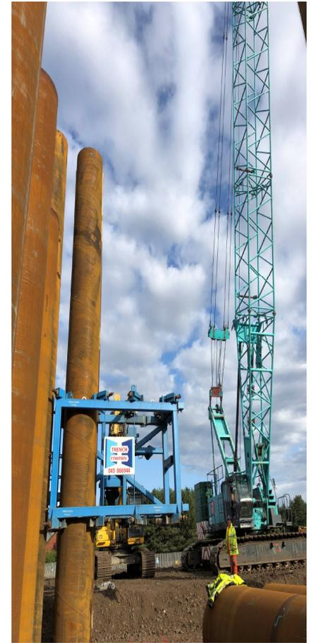
Once the combi tubes were pitched into position and are to vibro refusal, Trench control team impacted these tubes using CG300 impact hammer to initial refusal level. The main contractor then proceeded to core out the internals of each tube removing the debris from inside the tubes. TCL would then return to the cored tube and impact again to the design depth required.
