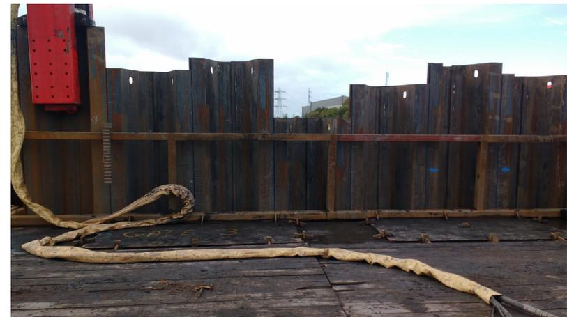
**Fished Product** – Once all aspects of our temporary & permanent elements had been installed the remaining anchor ties and concrete mass works could commence. Dewatering could begin and the dredging of materials to create the deep water berth could commence to completion.
