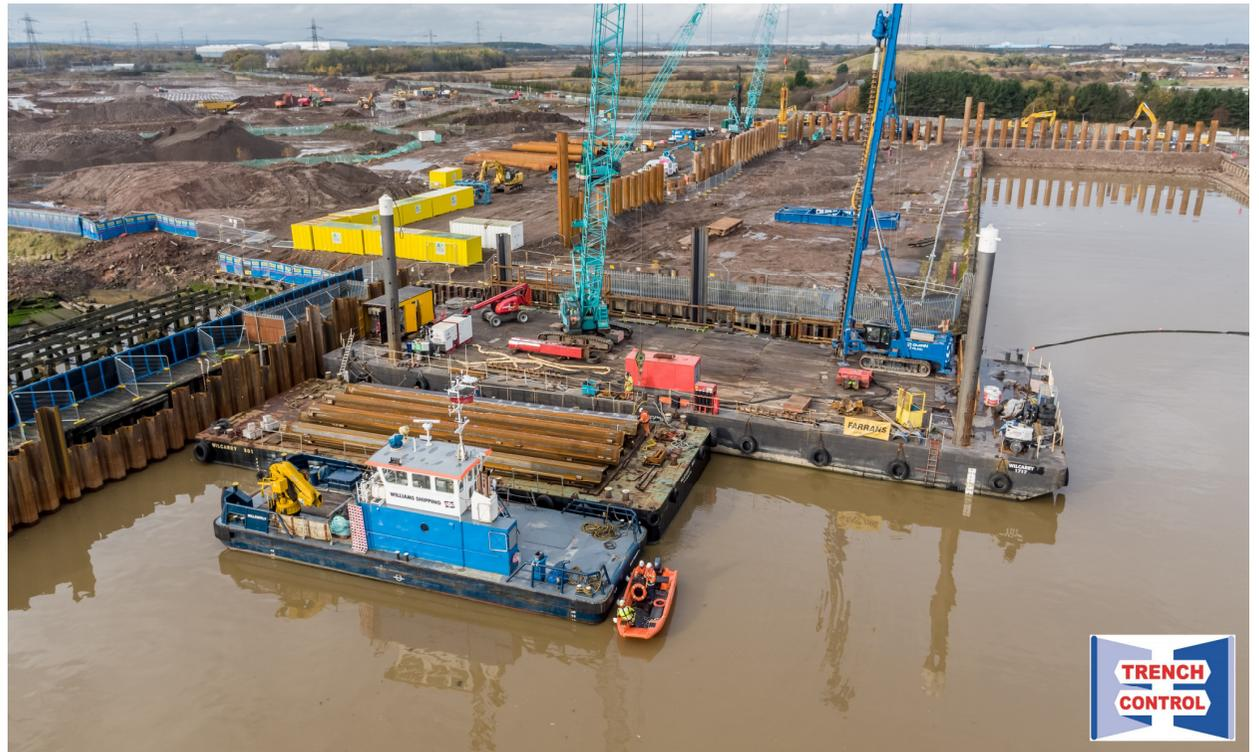
**Project Brief** – Following on from our successful installation of the south side deep water berth 9 & 10 at Montrose Harbour, Farrans Construction engaged Trench Control services again to utilise our hydraulic piling gate for a similar deep water berth in the north east of England. Northumberland Energy Park Phase 1 is to transform an existing dock into a deep water berth with jack up barge capabilities and is part of a strategic land development plan for the Blyth estuary.
