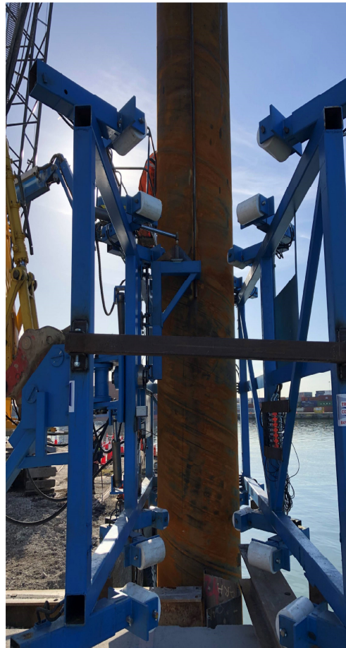
Hydraulic rollers guide tube
